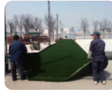
step1: Unroll the artificial grass carpet on the leveled foundation and leave them for a few hours for the natural extension.
