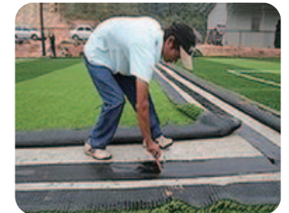
step6: Brushing glue on the tape and the edges of two grass carpet.
