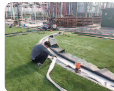
step7: Putting the white grass in the right place.
