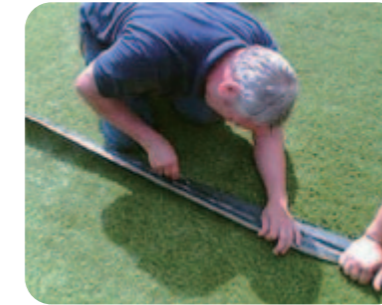
step2: Cutting the grass edges to fit the field size before you glue the seams.
