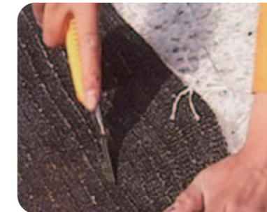
step5: Cutting the right size of the white grass.
