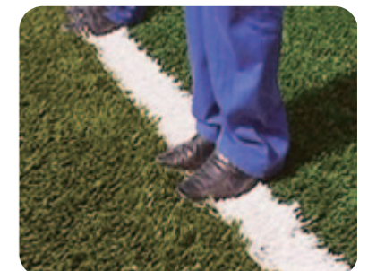
step9: Step the joint by foot or wooden hammer to keep the joint strong.
