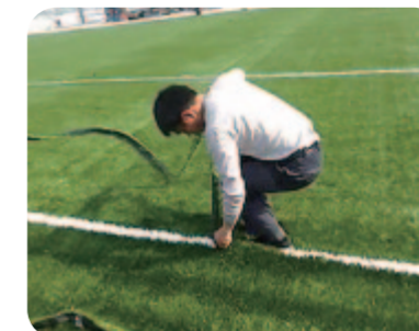
step8: Cutting the green grass which overlap on the white grass.
