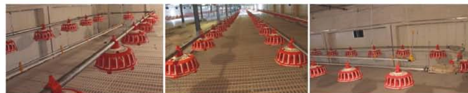
The layout for 3 circle chain-disc pan feeding system
